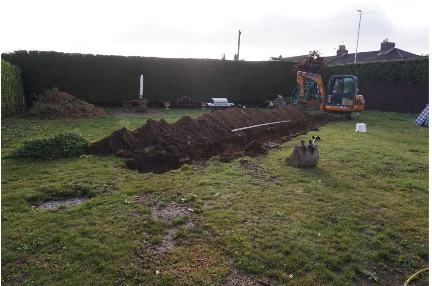
Plate 1: Looking SE at the site
