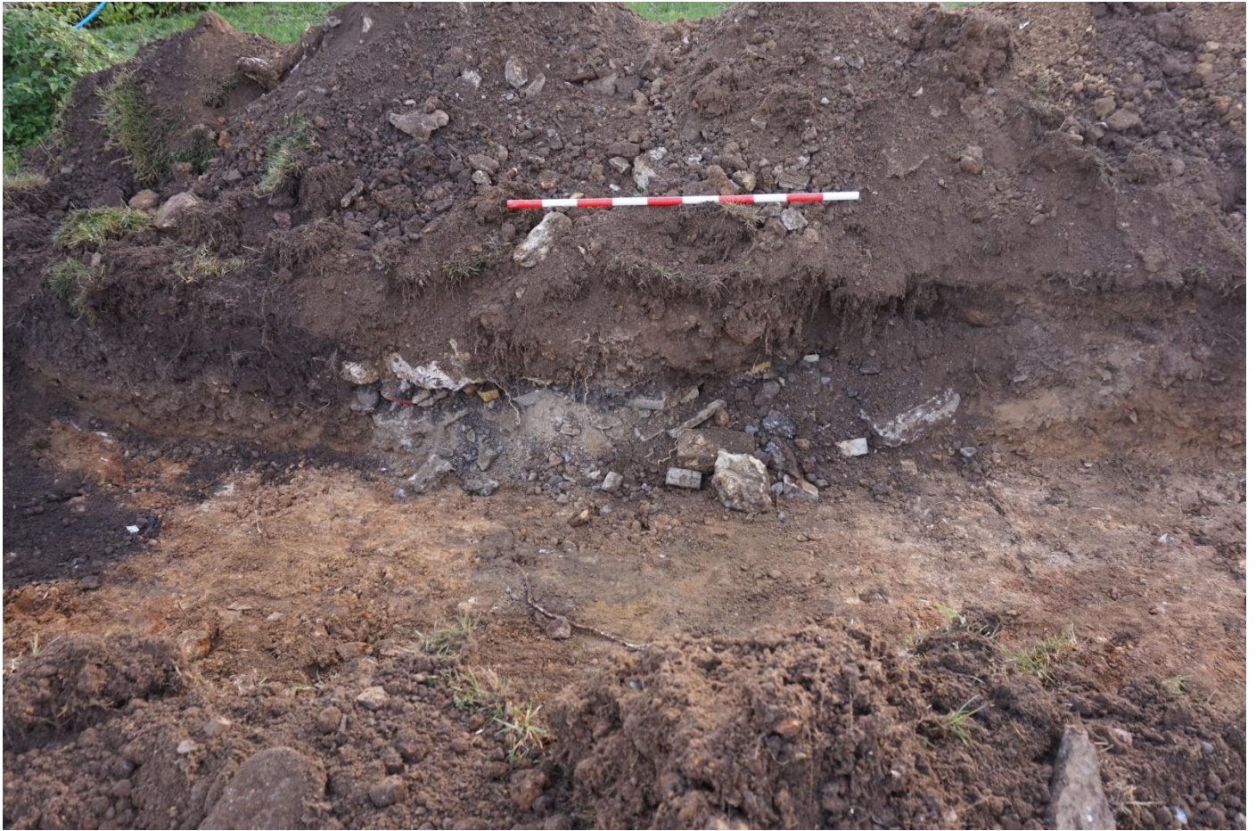
Plate 3: Looking ENE modern trench [104] backfilled with hardcore (105) and earth (106)
